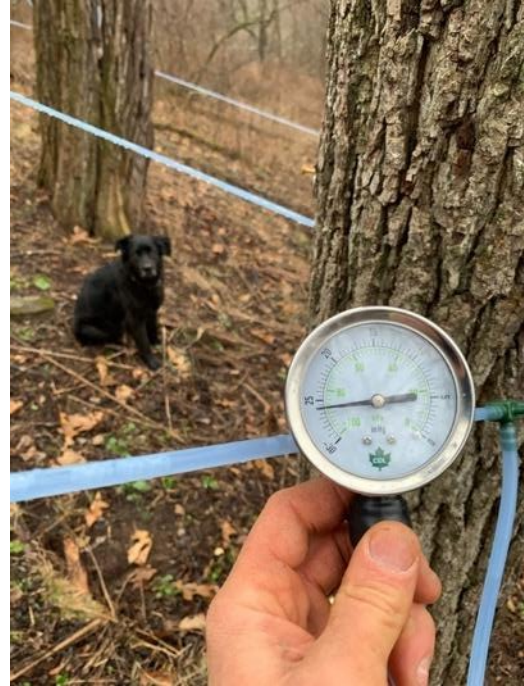
Figure 3: Vacuum gauge on a 3/16" gravity line
